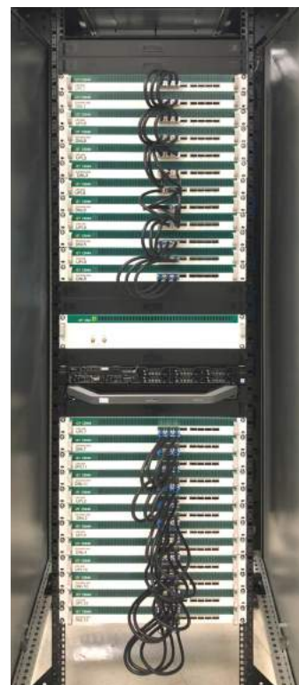
FIGURE 1: INSTALLATION OF MULTIPLE IZT C5040
